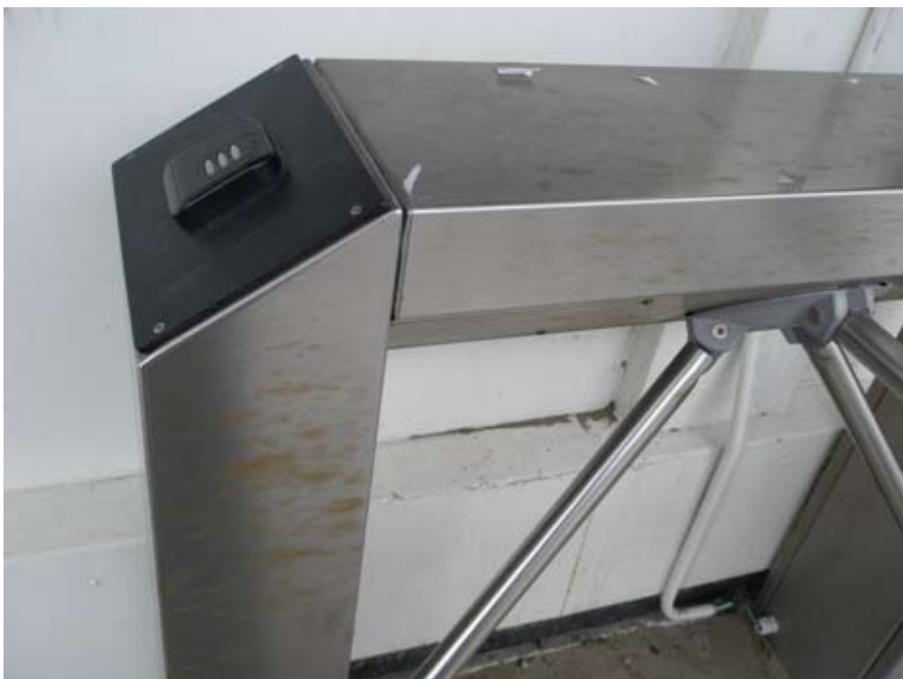
Fig. 2. RVS 316 access gate corroded by aerosols.
